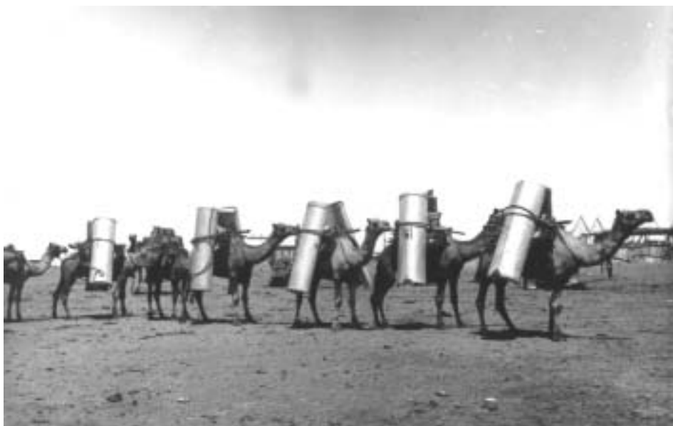
State developers. Carrying water pipes on the Nullarbor 1920s.
