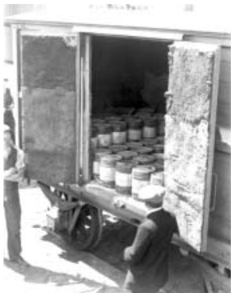
Explosives stored in a rail wagon at Dry Creek station near Cavan 1930s.
